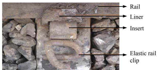
Fig.1. Atmospheric corrosion of rail base [14]
