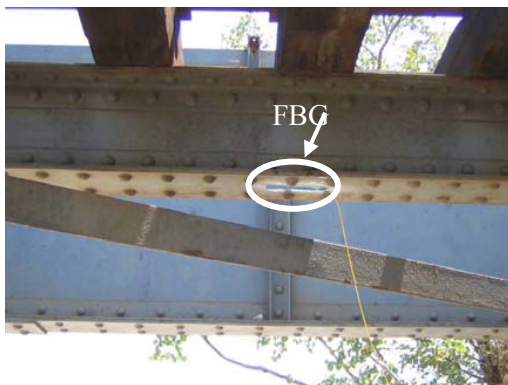
Fig. 8. FBG sensor installed on the beam section of the bridge
