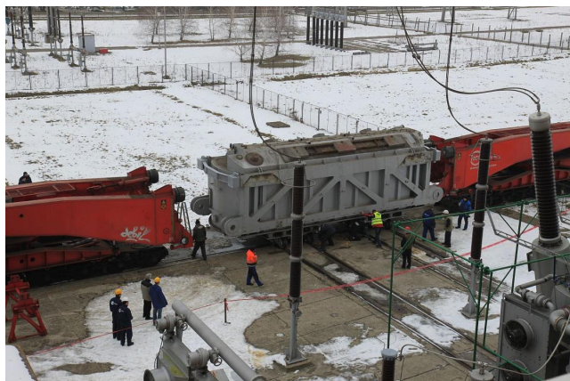
Fig. 4. 725 MVA transformer on the loading position for the “Schnabel” wagon at thermal power plant TENT B in Obrenovac
