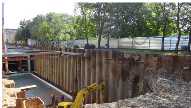
Fig.5. Tunnel in "Youth" complexe
