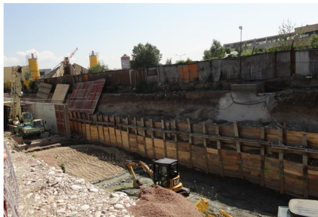
Fig.4. “Berlin wall” – Metal column whit wooden wall used to fortify the trenches.
