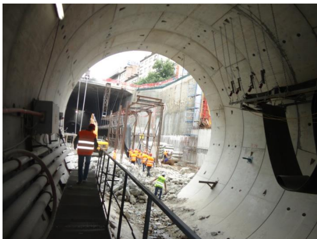
Fig.8. Tunnel made form tunnel boring machine
