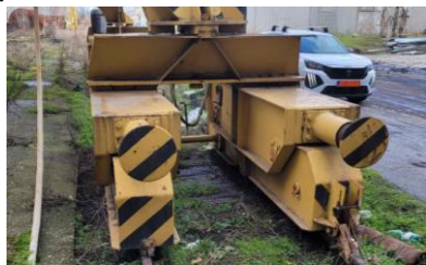
Fig.2. Existing condition of the crane track.
