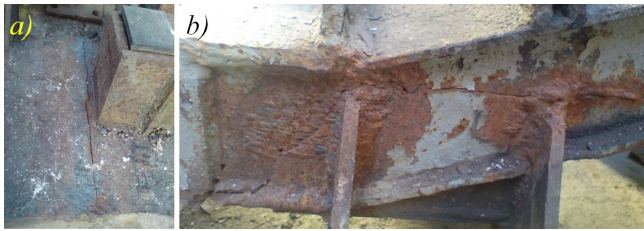
Picture 1. Occurrence of crack on the weld and developments in the vertical sheets.
