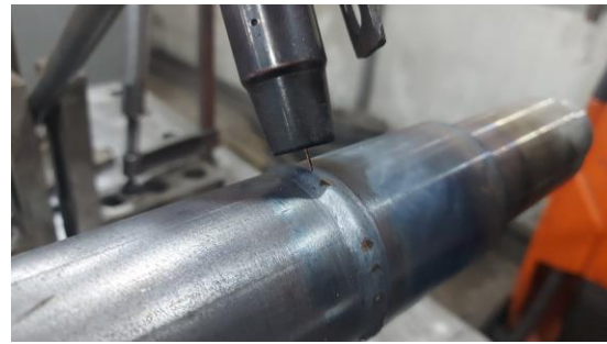
Fig.1. Welding of the sleeve and pipe joint
