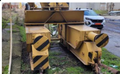
Fig.2. Existing condition of the crane track.
