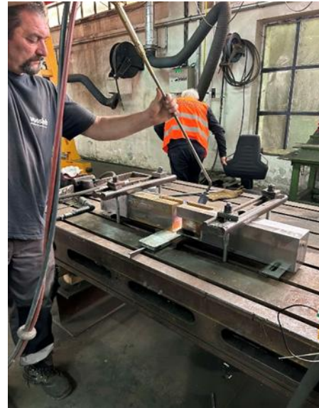
Fig 2. Preheating of the joint
